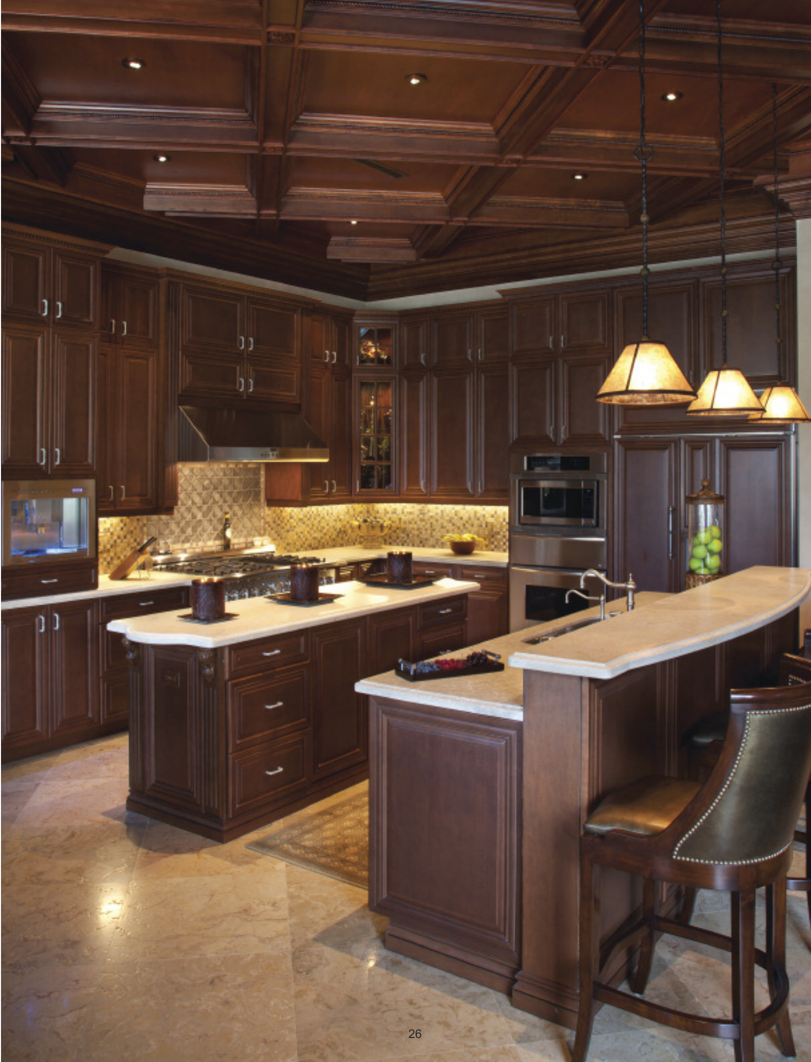
(LEFT) The original Kitchen drywall ceiling was completely covered to accommodate a custom wood box beam ceiling with new LED recessed lights resulting in a space totally transformed. Three custom mica and hand forged Iron pendants define the high bar.
